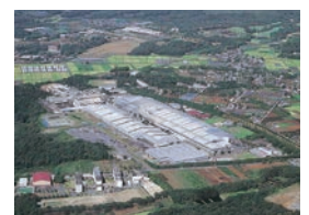
Copper tubing works (currently copper tubing works of UACJ Copper Tube Corporation)
