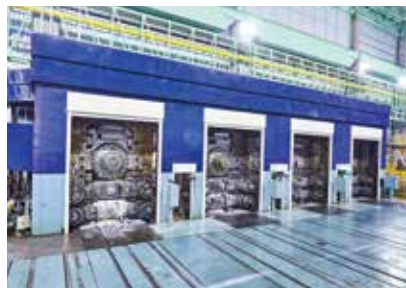
Four-stand hot finish rolling mill
