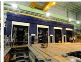
Four-stand finishing mill under construction
