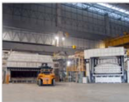
Making adjustments at melting furnace
