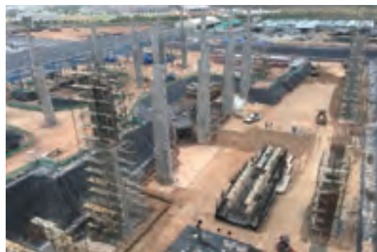
UACJ's aluminum casting plant under construction in Thailand
