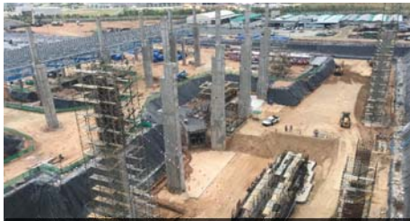
The third phase of construction of an aluminum rolling mill
