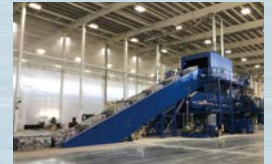
A scrap recycling furnace
