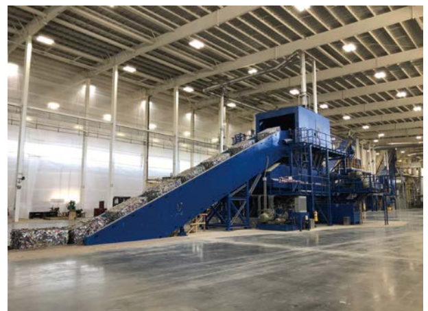
A scrap recycling furnace at Tri-Arrows Aluminum Inc.
