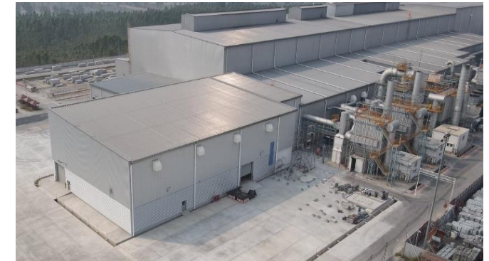
UATH: New scrap melting furnace
