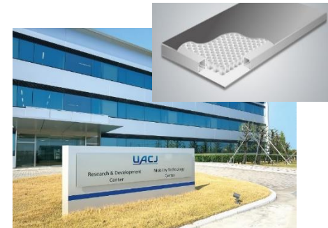
UACJ R&D Center exterior and eaves
