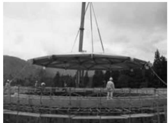
Fig. 7 Lifting up of the Dome-Truss cover over the tank.
