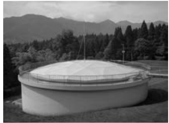
Fig. 5 Appearance of the service water tank with aluminum Dome-Truss cover built in Nikko.
