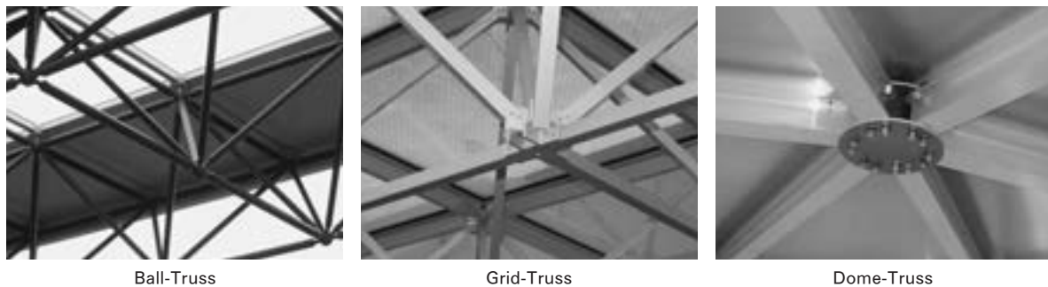
Fig. 1 Various types of System-Truss.
