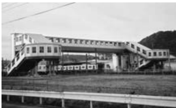
Fig. 2 Nishikaratsu Station overbridge of JR Kyushu.
