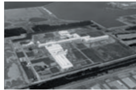
Fukui Works at the time of completion
