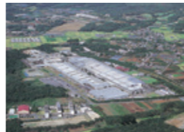
Copper tubing works (currently copper tubing works of UACJ Copper Tube Corporation)
