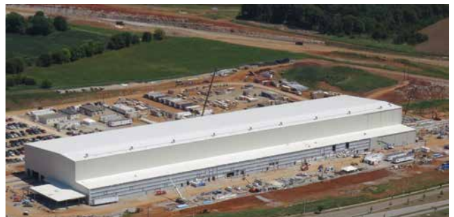
Plant construction is moving ahead on schedule with a view to commencing operations in fiscal 2016
