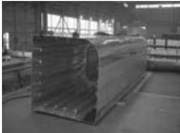
Fig. 6d Fabrication of girder units.
