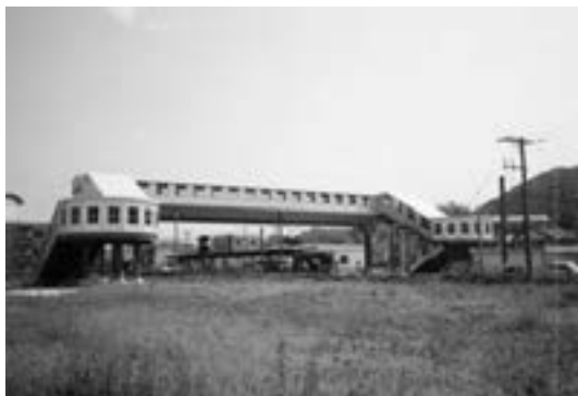
Fig. 3 Nishikaratsu Station overbridge.
