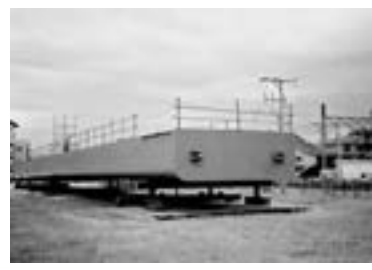
Fig. 6f Field assembly near the site.
