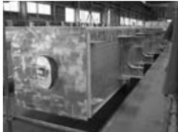
Fig. 6e Fabrication of girder block.
