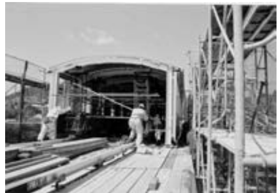
Fig. 19 Sliding the shelter on the bridge.
