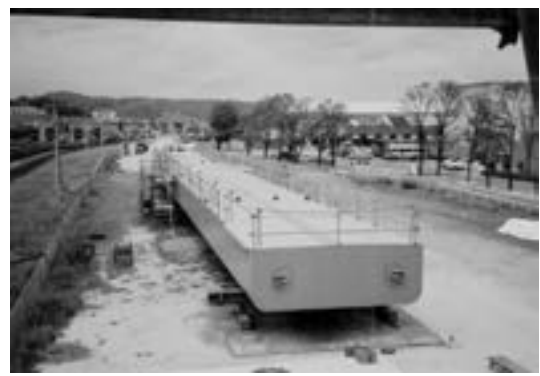
Fig. 16 Field assembly near the site.
