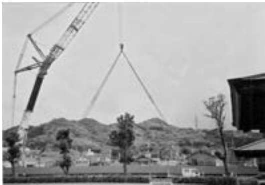
Fig. 18 Lifting by 360tons truck crane.
