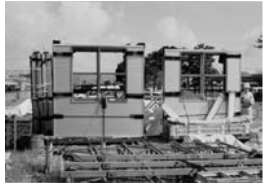
Fig. 15 Units of the wall.
