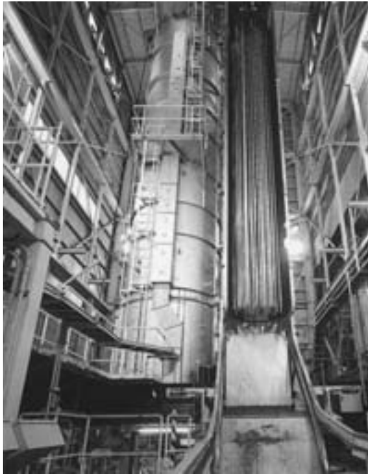
Fig. 35 Vertical furnace with quenching equipment
