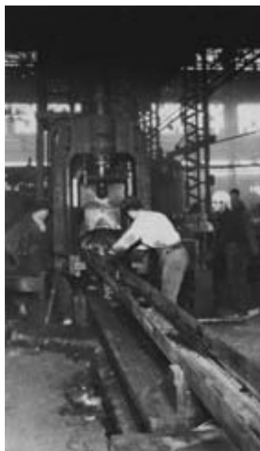
Fig. 18 Horizontal hydraulic pressure extrusion press for shapes (from 100 Years of Working with Copper and Aluminum, 1897-1996 , Sumitomo Light Metal, 1997)
