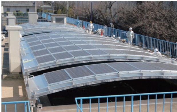
図2 浄水場覆蓋 Fig.2 Aluminum cover for water filtration plants.
