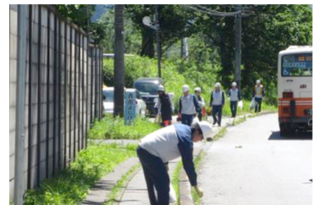
Cleaning up near the Nikko works
