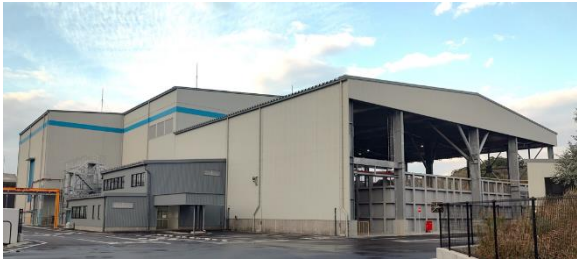
UACJ Yamaichi Aluminum Can Recycling Co., Ltd. (at Fukui Works) New used beverage can processing facility exterior
