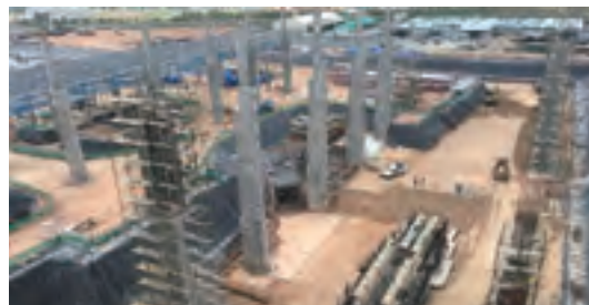
建設中の casting building
