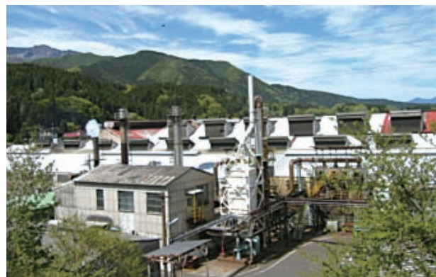
燃料転換後 (After fuel switching)
