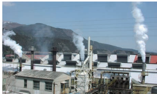
燃料転換前 (Before fuel switching)
