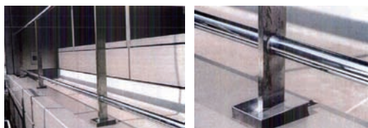
図1 もらい錆の事例 Fig.1 Example of contagious rusting.
