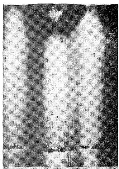
**Photo. 9** Transverse overlapping zone of aluminium corrugated sheet with the other one. Corrosion attacks are not appeared in overlapping zone but the interface is remarkably corroded. Unweatherside.
