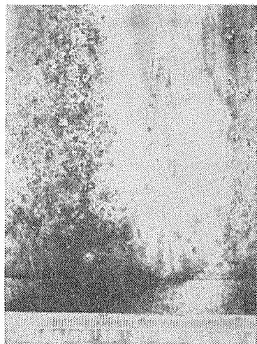
**Photo. 19** Transverse overlapping zone of aluminium corrugated sheet. Weatherside. Remarkable corrosion attacks are appeared in overlapping zone.
