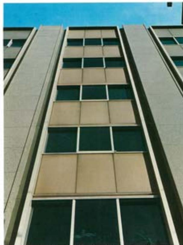
Fig.8 Appearance of building after 10years exposure.
