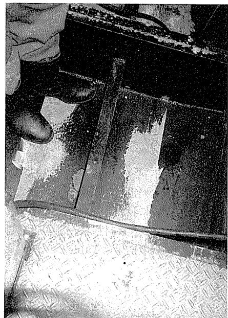
Fig. 3 Corrosion appearance on the bottom.
