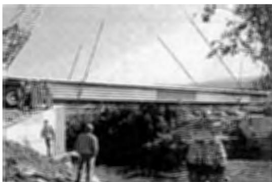
Fig. 11 Installation of first aluminium road bridge in Norway<sup>20)</sup>.
