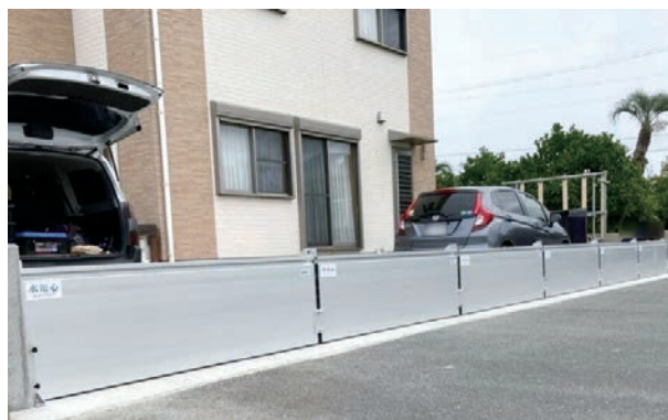
Fig. 6 Example of installation on a residential parking space with 14 meters width flood barriers.
