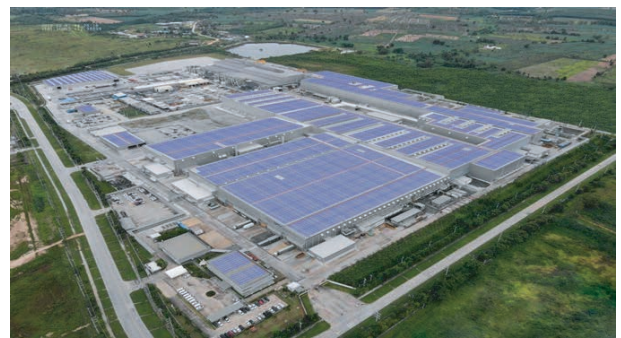
Fig. 11 Solar power generation system at UATH (Rayong Works).
