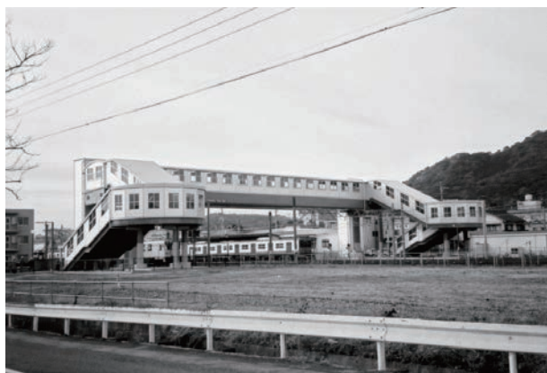
Fig. 3 Nishikaratsu Station over-bridge of JR Kyushu 1) .
