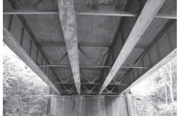
Fig. 29 Bridge construction manufactured by MIG welding 50 years ago.
