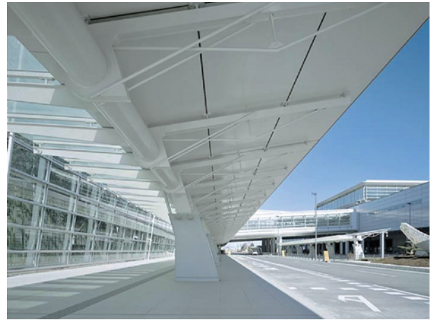
Fig. 3 Honeycomb panel eaves of the Chubu Centrair International Airport.
