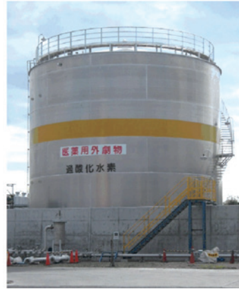
Fig. 6 The Aluminum Storage Tank for high-pressure hydrogen peroxides.
