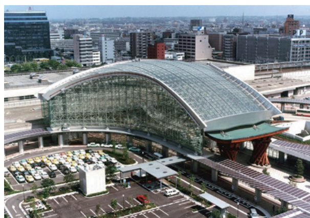
Fig. 1 The Motenashi Dome of JR Kanazawa Station, which is the largest space truss structure roof made by aluminum alloys in Japan.
