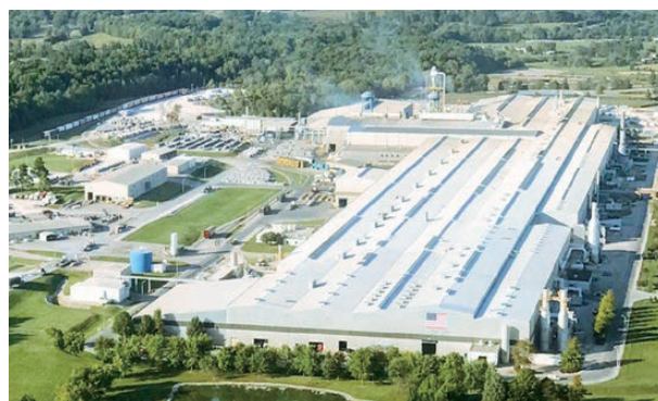
Fig. 1 Logan Aluminum which is Al sheet production plant of TAA.
