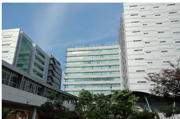
Fig. 1 Innovation Cluster II building.
